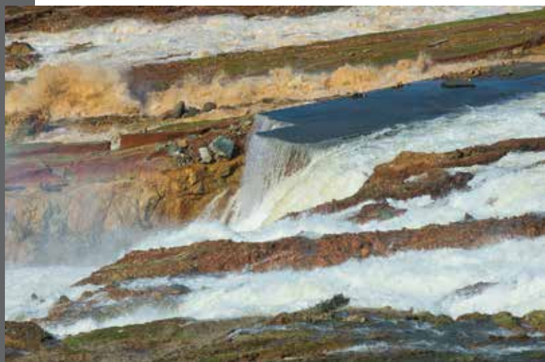
Emergency Spillway Flows and Erosion. Water flows over the Emergency Spillway for the first time on Feb. 12, 2017, eroding gullies and destroying a roadway. Source: Kelly M. Grow, DWR.
