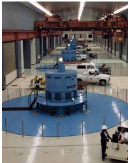
Oroville Hydropower Facilities. Located beneath Oroville Dam, the Edward Hyatt Powerplant contains six units, three to pump water and three to generate power for the operational needs of the DWR facility. Source: DWR. Ronald B. Robie Thermalito Pumping-Generating Plant, located at the Thermalito Afterbay, at sunrise 11/23/12. Source: Florence Low, DWR.
